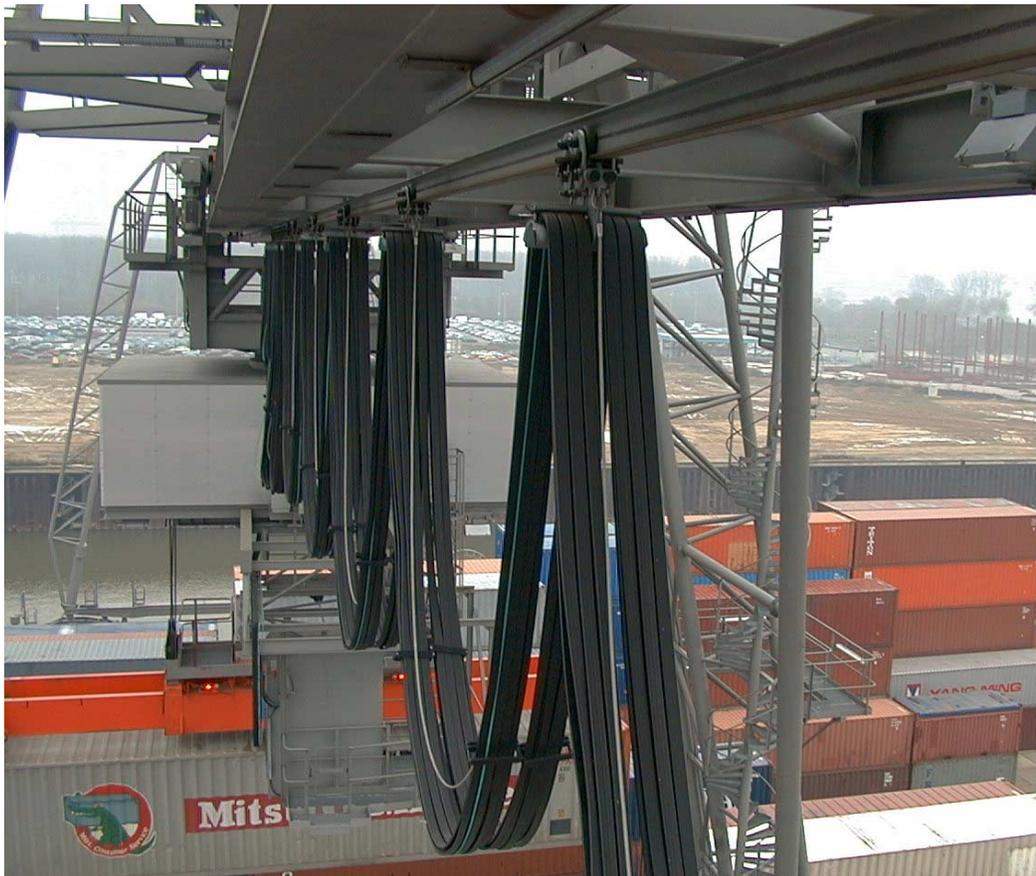
Figure 4-11 Use of the PROFIBUS Cable for Festoons
